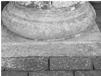
TUSCAN COLUMN RENOVATION TUSCAN SAND STONE BASE AFTER REMOVAL OF COATING AND MODERN PAINTS. LOCAL SANDSTONE WAS USED TO CARVE THE ORIGINAL BASES.
