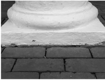
TUSCAN COLUMN RENOVATION STONE BASE BEFORE REMOVAL OF PATCHING AND COATINGS
